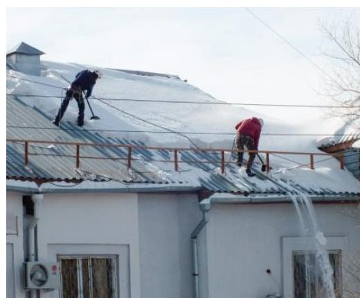
**Figure 4. Mechanical removal of snow from the roof of the house**
