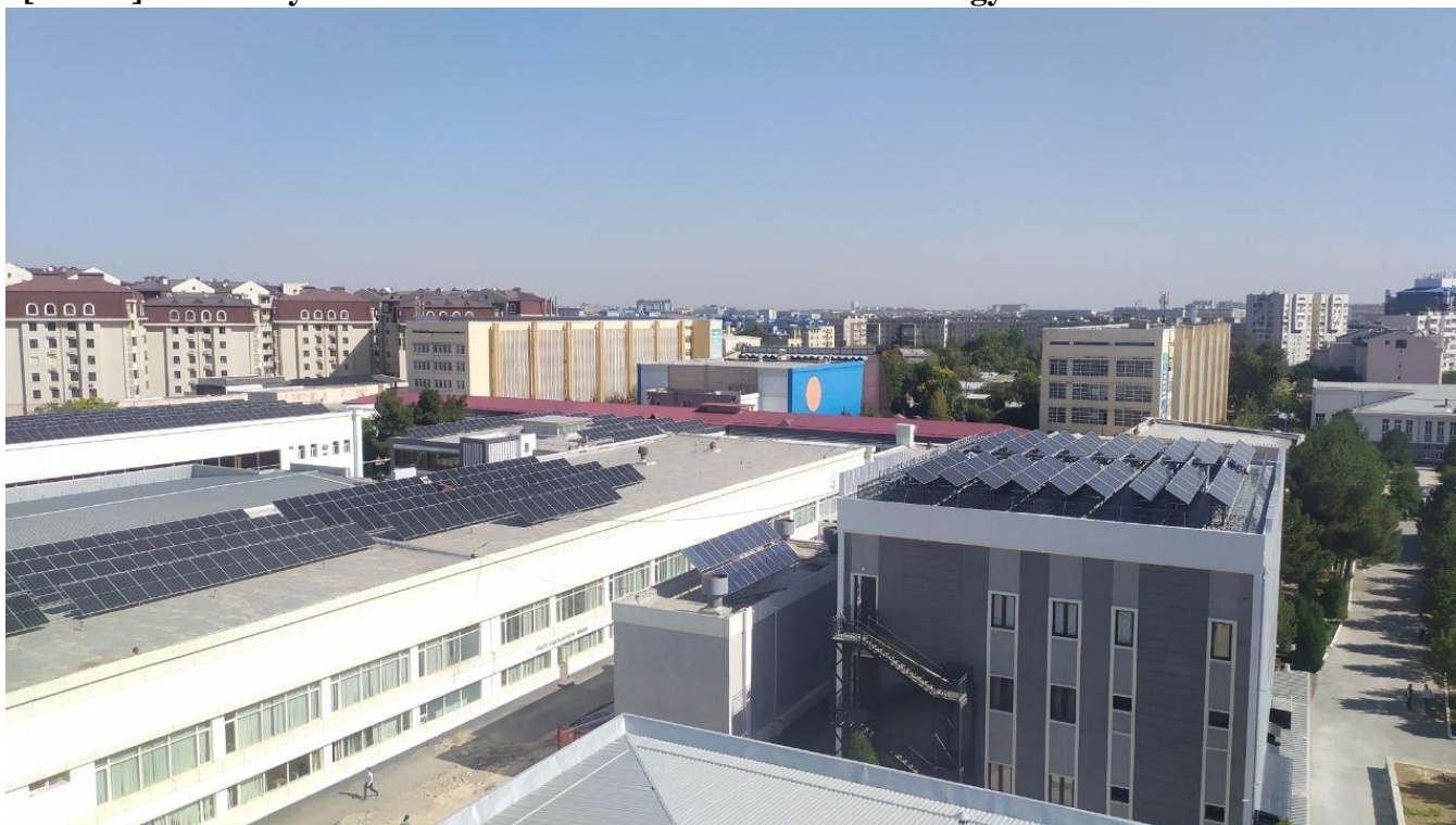
Roof Mounted Solar Panels (“TIAME” NRU)
