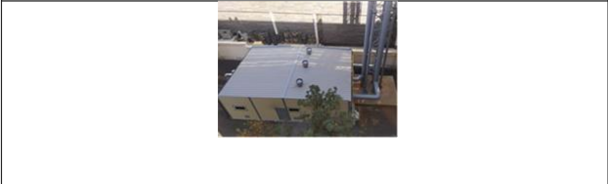
Individual campus heating system to reduce natural gas (Heating system based on electric heats and use solar energy )
